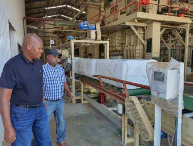
The Team observing the operation of electrified Press
