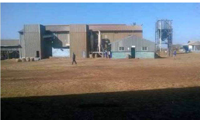
Ginnery Plant at Big Bend
